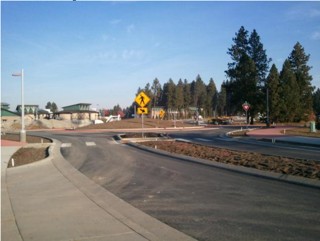
Northern boundary of request adjacent to WWTP:
